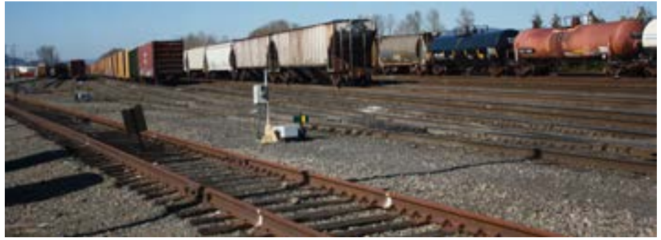
Longview Switching Yard
